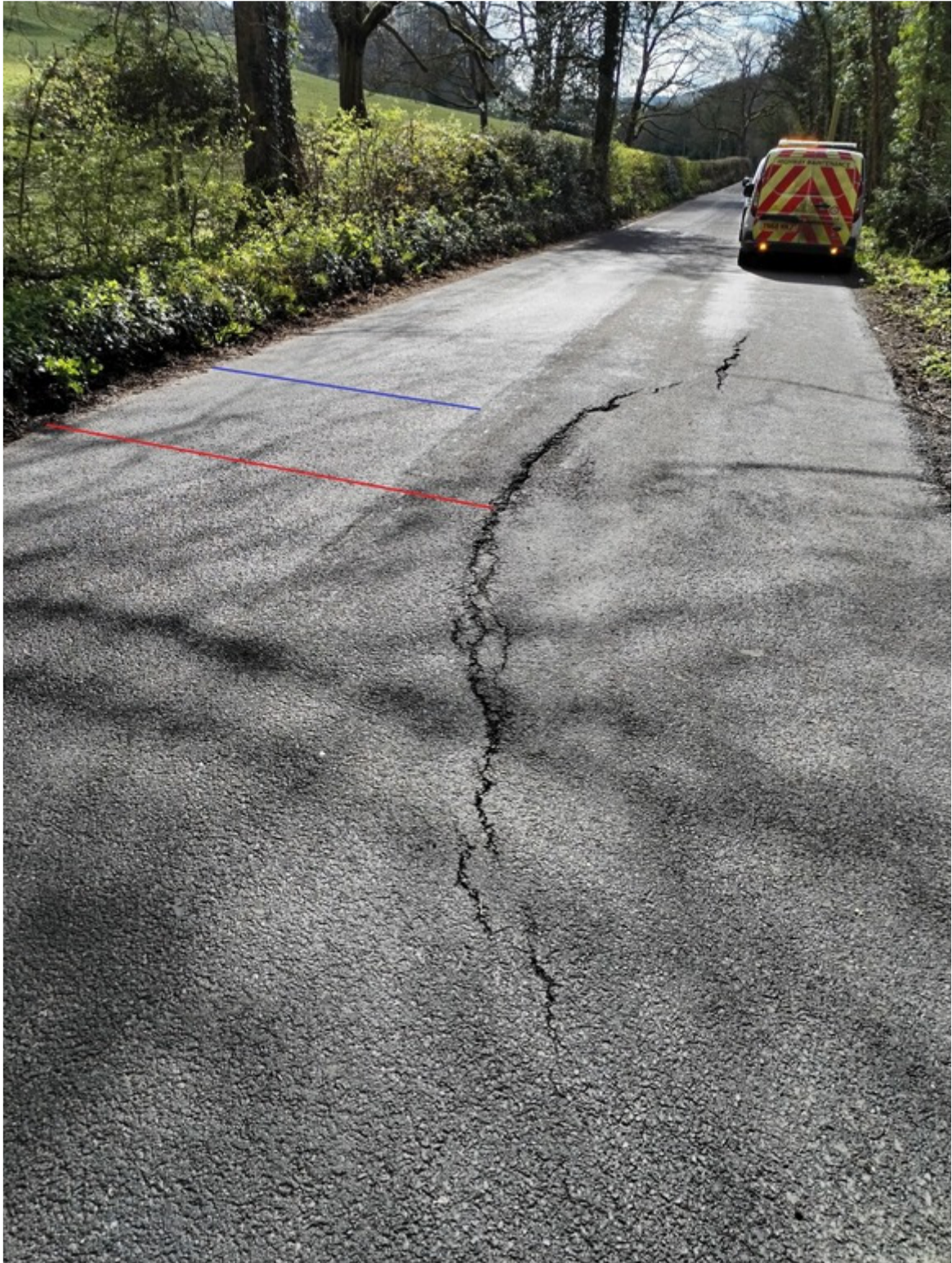
Lea Road inspection photo
